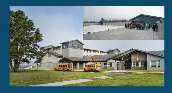
The first tsunami vertical structure in the United States: Ocosta Elementary School, Westport, Washington. The building is designed to withstand an earthquake and has a flat roof over the gym to accommodate up to 1,000 students and community members from a resulting tsunami.
